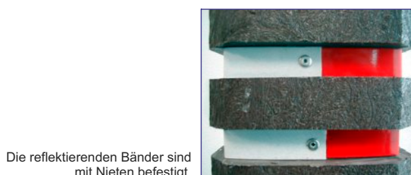
the reflective strips are mounted with rivets
